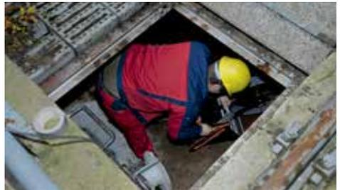
*Camera inspection for identifying the extent of damage*
